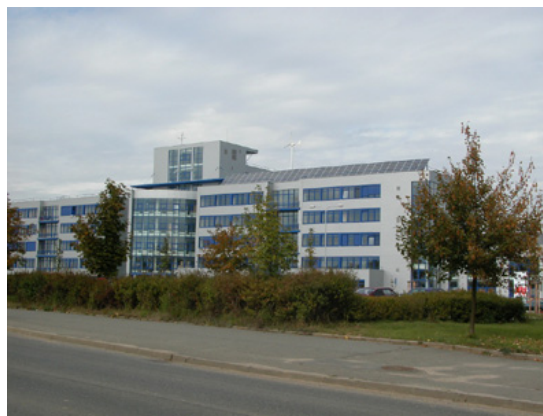
Fig. 1 20 kW p photovoltaic system
